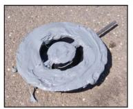
5. Press the base down firmly on the road surface until epoxy appears around the edge. The arrow must face traffic.
