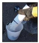
4. Apply epoxy evenly to the bottom of the base; including the middle section.
