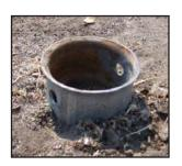
6. Insert the post and align the holes in post with the holes in the anchor. Use a bolt and lock nut to secure the post to the anchor.
